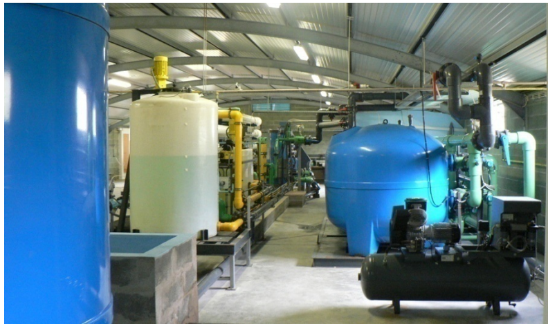
Technical tour auxiliary equipments
