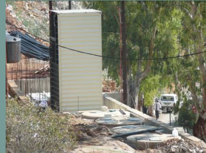
Type: wind-vapour compression Location: Symi, Greece Capacity: 20m 3 /h Year of installation: 2009 Still in operation: yes Usage: drinking water
