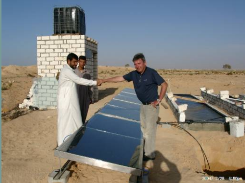
Type: F8, 8 modules 1.25 x 1.25 m 2 Location: Alexandria /Egypt Capacity: average ca. 50-60 l/d Year of installation: 2004 Still in operation: yes Usage: drinking water for desert camp
