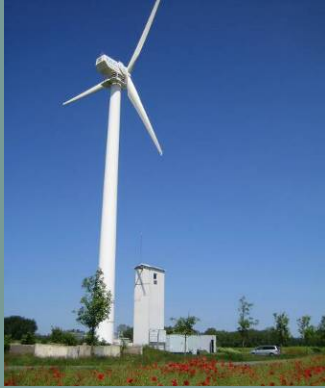
Type: wind-vapour compression Location: Rügen Island, Germany Capacity: 15 m 3 /h Year of installation: 1995 Still in operation: yes Usage: drinking water
