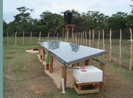
Type: F8, 6 modules 1.25 x 1.25 m 2 Location: Cuba Capacity: average ca. 40 l/d Year of installation: 2006 Still in operation: yes Usage: drinking water for a family
