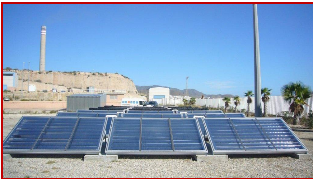
100 m 2 MAXI collector field installed in a demonstration desalination plant in Carboneras, Spain (project MEDESOL)
