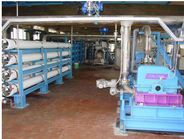
Reverse osmosis plant in Porto Santo
